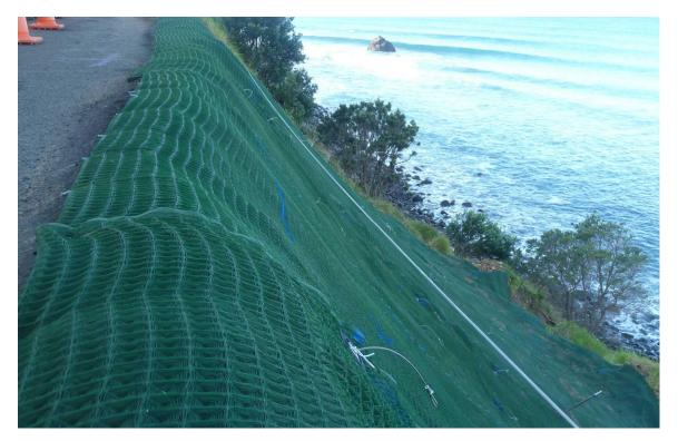
Figure 4.1B. Pyramat HPTRM Shoulder/Embankment Installation Credit: Cirtex Civil
