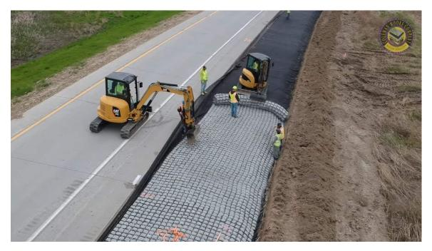
Figure 4.1A. Flexamat ACBM Installation Along Roadway Shoulder Prone to Overtopping Credit: Flexamat/Coleman Moore Company
